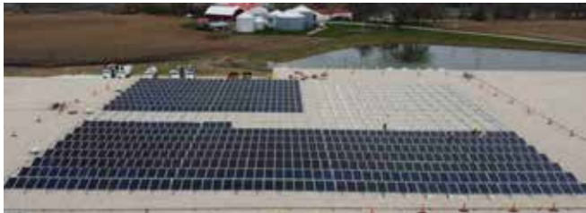
Alamo Group’s Super Products vacuum truck production facility in Mukwonago, Wisconsin began producing renewable electricity from their rooftop Solar PV array in April 2021. This system is anticipated to provide about 400,000 kWh of renewable power annually, or about one third of this facility’s electric power consumption.
